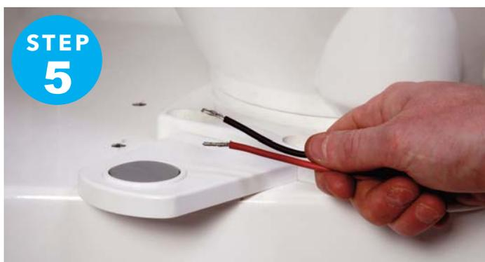
The next step is to connect to the power supply. The boat's positive feed needs to be connected to the red lead, and the negative feed to the black lead. Always ensure that a suitable size circuit breaker and wiring is used and consult an electrician if you are unsure of this. The electric toilet is almost operational.
